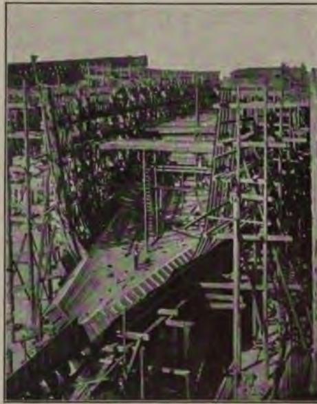
Building a steel ship at Newport News.
